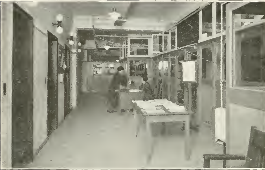
Hall and information desk on the fifteenth floor.
